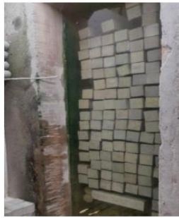
Figure 3. Curing of concrete blocks.
